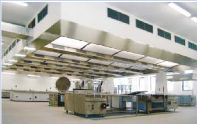
• Army catering facility Vyškov •
